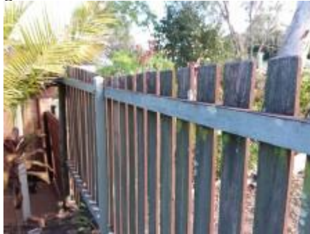
Weathering and slight wood rot to garden Timbers
