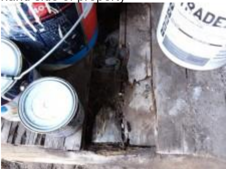
Wood rot to wooden fence line to left-hand side of property
